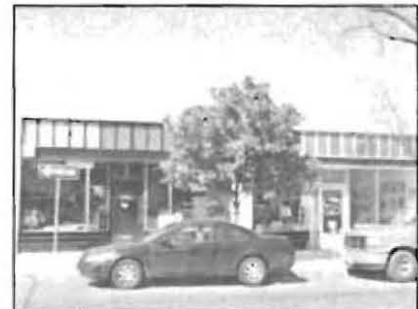
Shopfront on a One-Story Commercial Block
