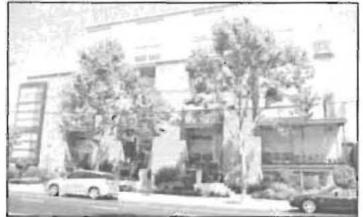
Modern Stacked Flats with Stoop Frontage
