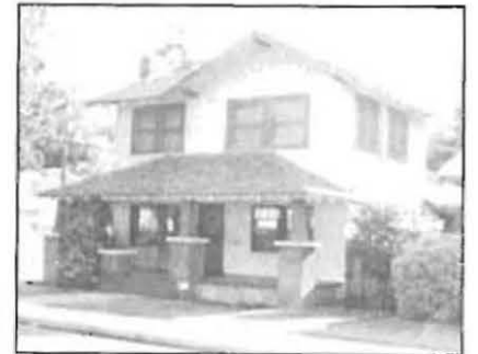
Porch on a Two-Story Front Yard House
