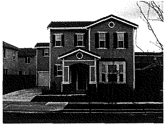
Home with a single-car width driveway that widens to a two-car apron in front of recessed garage.
