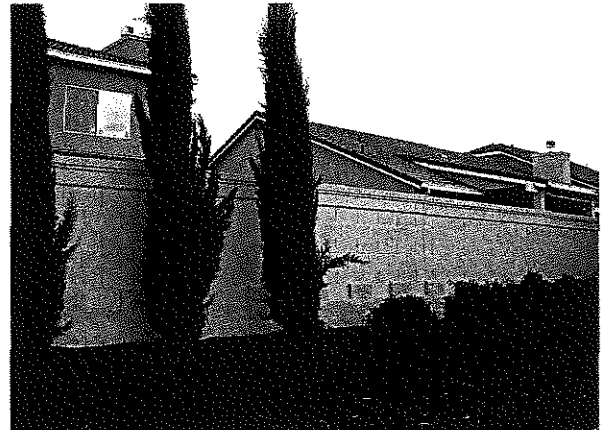
Encouraged: walls architecturally integrated with adjacent buildings; landscape buffer between wall and sidewalk/street.
