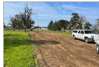
Fine Grade of sod at golf course
