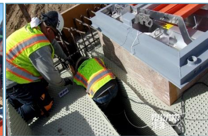
Installation of HDPE Line at Wet Well Deck
