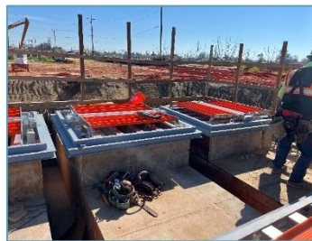
Installation of Hatches at Wet Well Deck
