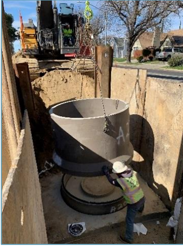
Placement of SSMH components at intersection of Tuolumne and Neece
