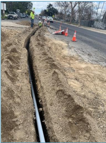
Installation of 2-inch fiber optic conduit on Tuolumne
