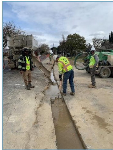
Slurry backfills at fiber optic trench on Tuolumne
