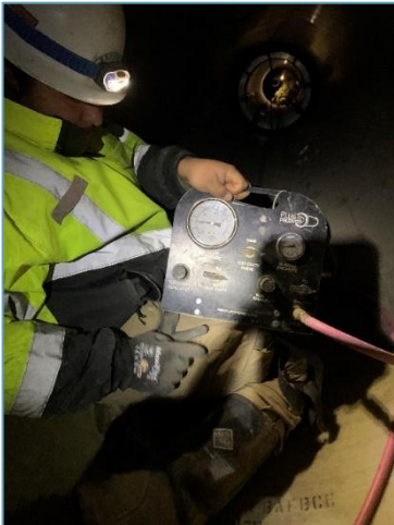
FRPMP joint air pressure testing operations
