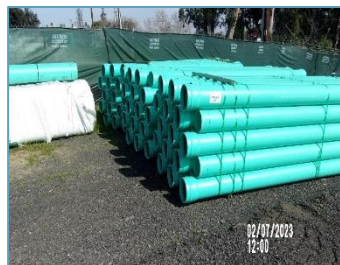
8-inch Sewer Pipe
