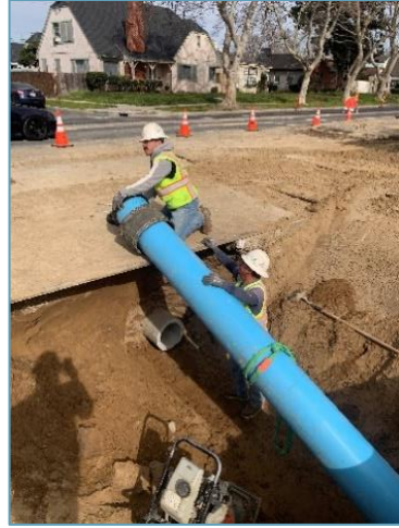
Replacement of pipe prior to completing trench backfill
