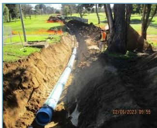
18-inch pipeline through Golf Course
