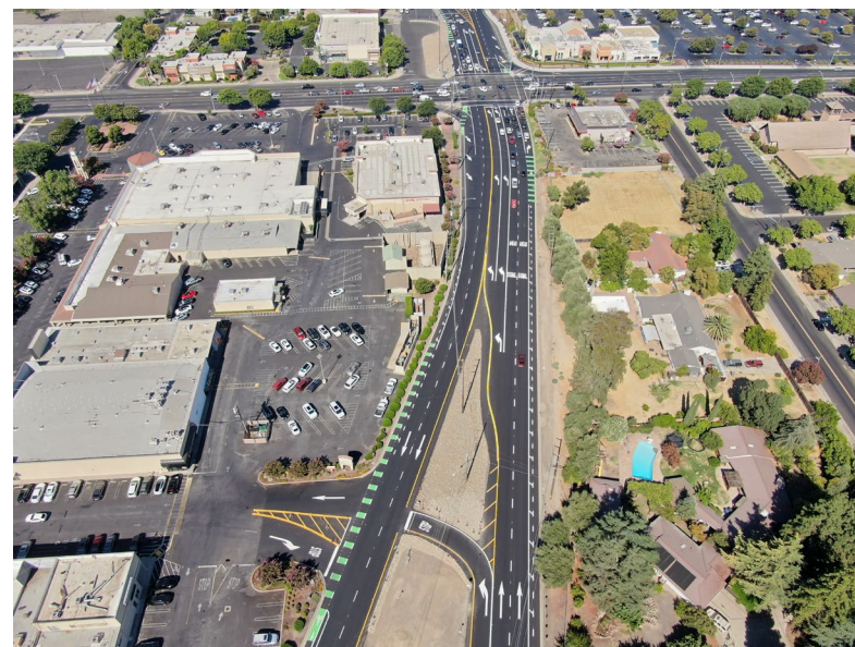
Briggsmore Avenue Rehabilitation Project
