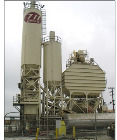
Light industrial business in Area 1
