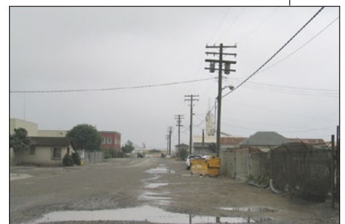
Streets such as Culpepper Avenue could benefit from design guidelines that encourage streetscape improvements.
