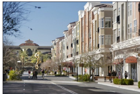
Vertical mixed-use development with a residential component in Henderson, Nevada
