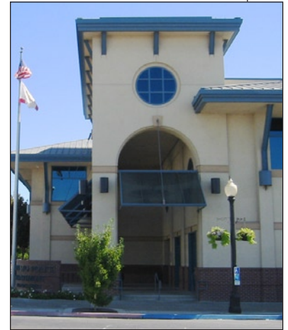
Existing Police Headquarters at 10th and G Streets
