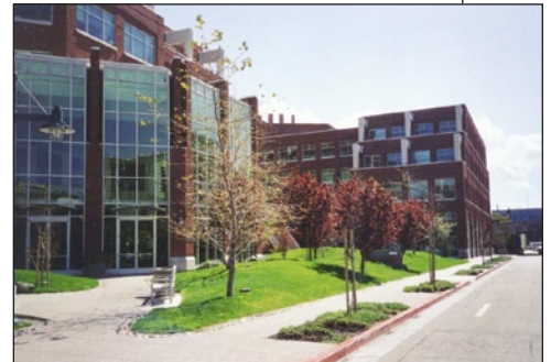
Development such as Emery Station in Emeryville, California, could be targeted for Area 2.
