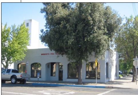
Existing Fire Administration Building at 11th and F Streets
