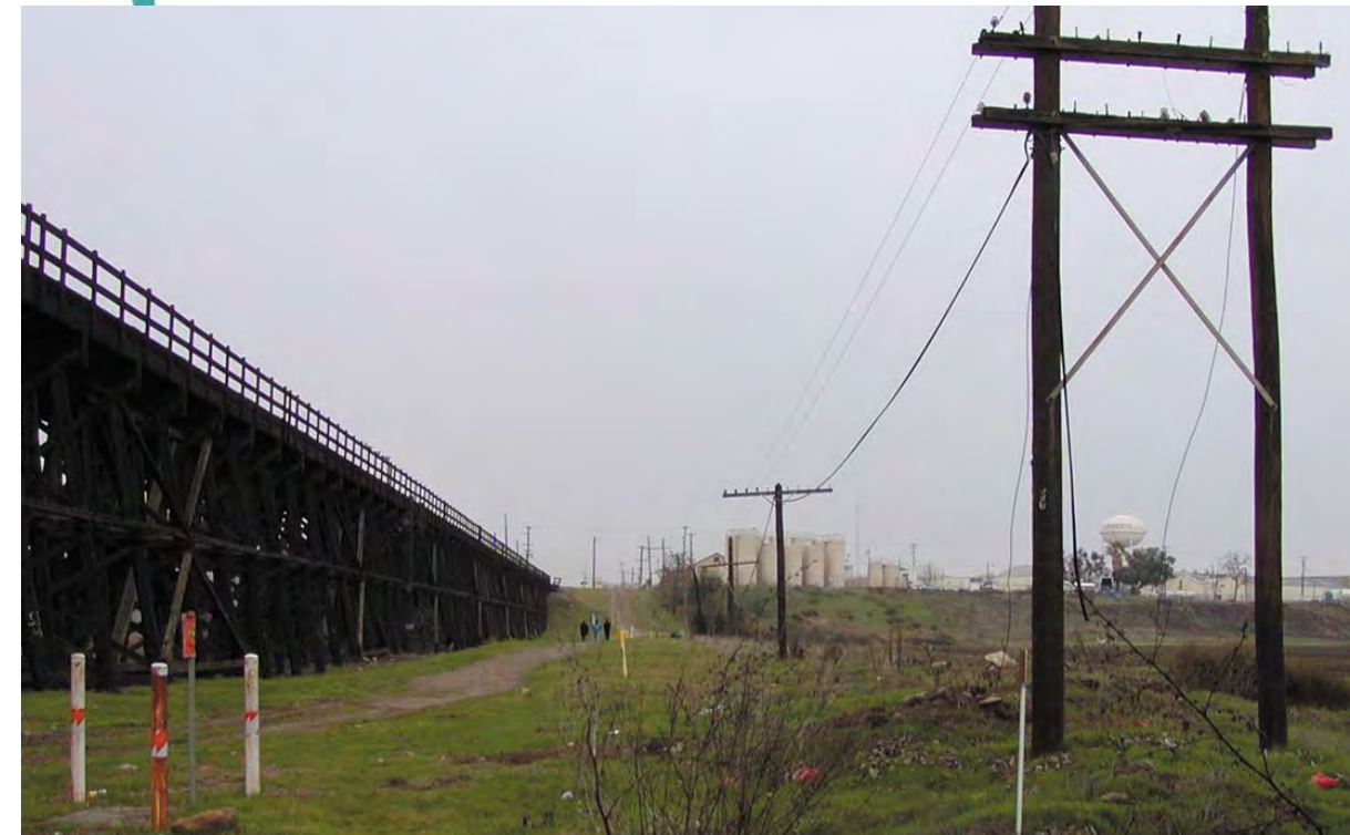
2004 Source: HDR Engineering Figure 35. Several utility lines were identified and mapped for the Precise Plan in order to prevent design and infrastructure conflicts. Utilities found included electrical, water and sewage, as well as telephone, fiber optics and a petroleum line.
