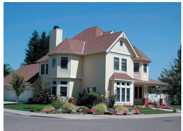
Example of four-sided architecture and design treatments: veneer wrapping, window sills, and decorative bracing along roofline.
