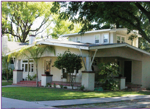
Left: Figure II-12 The additional setback of the second story (stepped back) helps to reduce the apparent massing and scale of the house.
