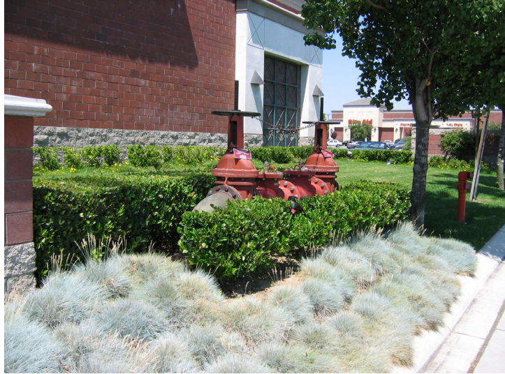
Figure 111 -- Utility lines screened by landscaping
