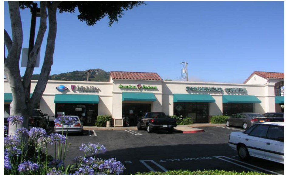
Figure 30 -- Wall signs should consist of individual letters compatible with the form and character of the building.
