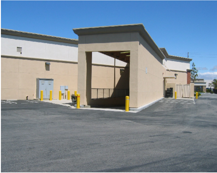
Figure 69 -- Loading area completely enclosed with same materials used for building
