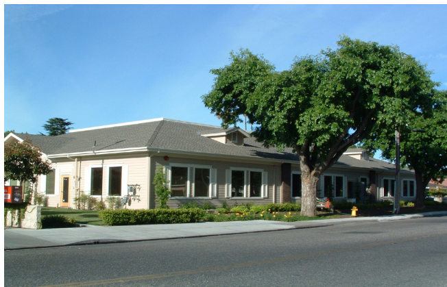
Figure 10 -- 200 B Roseburg Avenue
