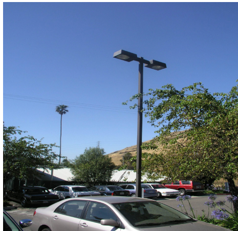
Figure 49 -- Lighting for parking areas should be designed to confine the light to the site.
