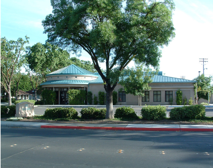
Figure 13 -- 205 W. Granger Avenue
