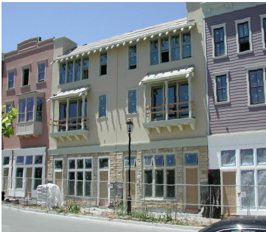
Figure 26 -- Window replacement should be consistent with adjoining buildings
