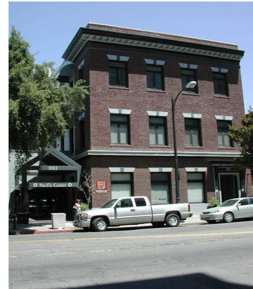
Figure 5 -- The Pacific Center, 1012 11th Street
