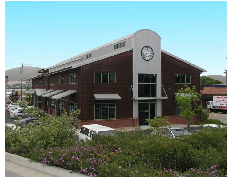
Figure 112 -- An example of an attractive metal building
