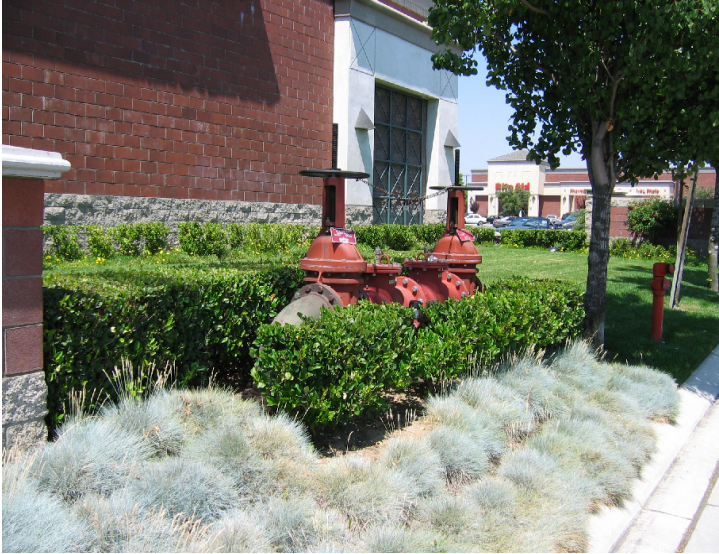
Figure 45 -- Utilities screened by landscaping
