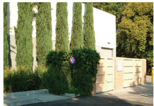
Service/loading area is effectively screened using decorative walls and vegetation.
