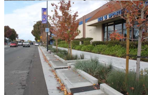
Consider ways to integrate various on-site LID design techniques, such as green roofs, stormwater retention areas and swales to reduce drainage costs.
