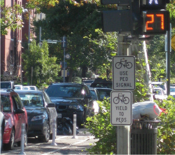
A bicycle signal head at a signalized crossing creates a protected phase for cyclists to safely navigate an intersection.
