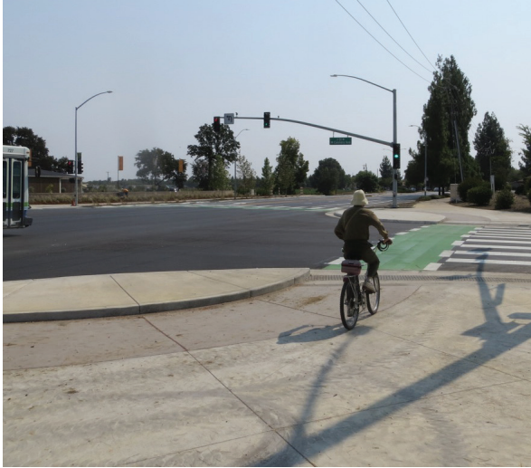
Protected intersections feature a corner safety island and intersection crossing markings.
