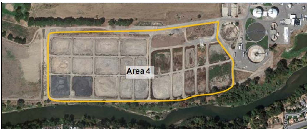
Figure 3-2 Condition Assessment Area 4 – Sludge Drying Beds
