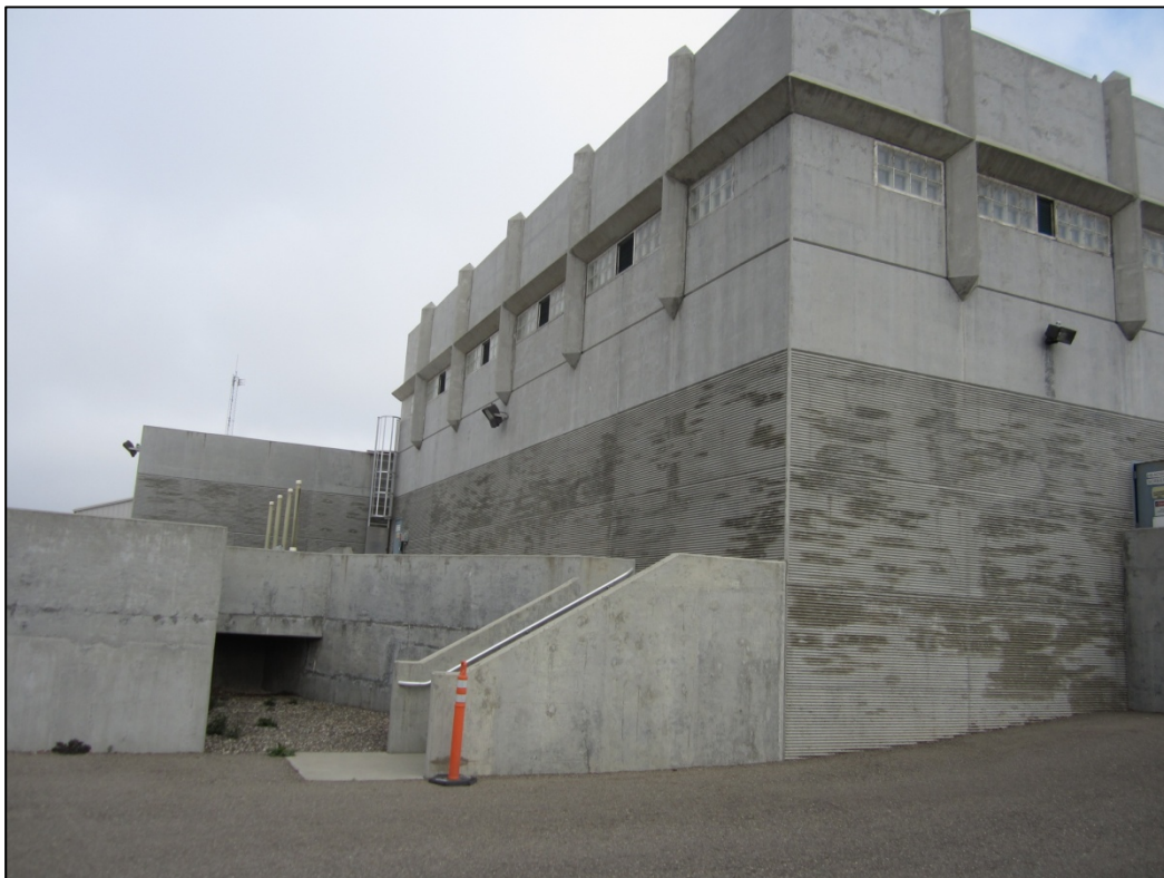
Figure 3-4 Headworks grit tanks and Parshall flumes (looking north).
