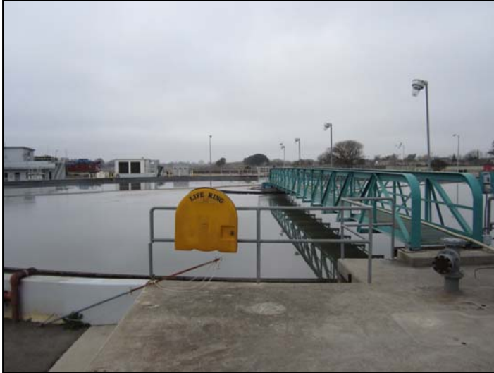
Figure 3-6 Primary Clarifier No. 1
