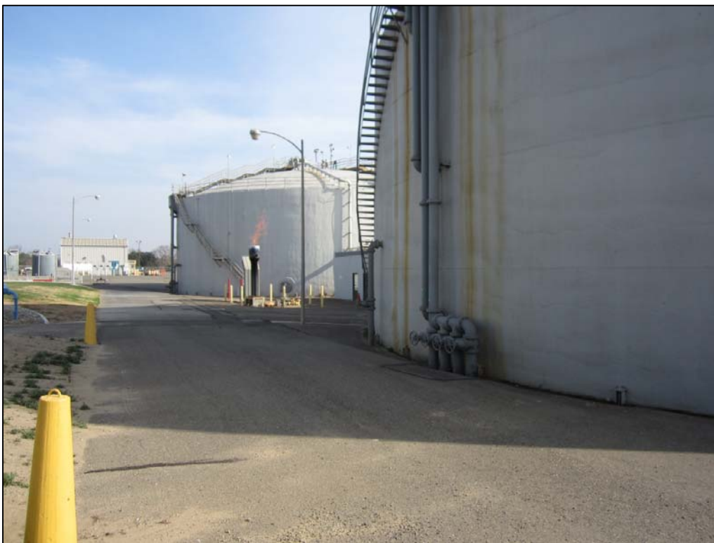
Figure 3-15 Primary Anaerobic Digesters No. 1 and No. 2
