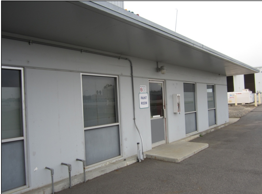
Figure 3-14 Picture of Paint Booth inside old Chlorine Building
