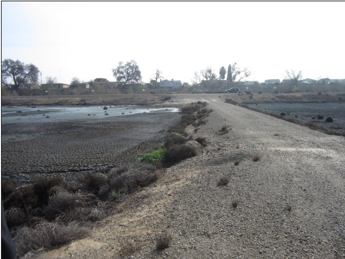
Figure 3-18 Sludge Drying Beds
