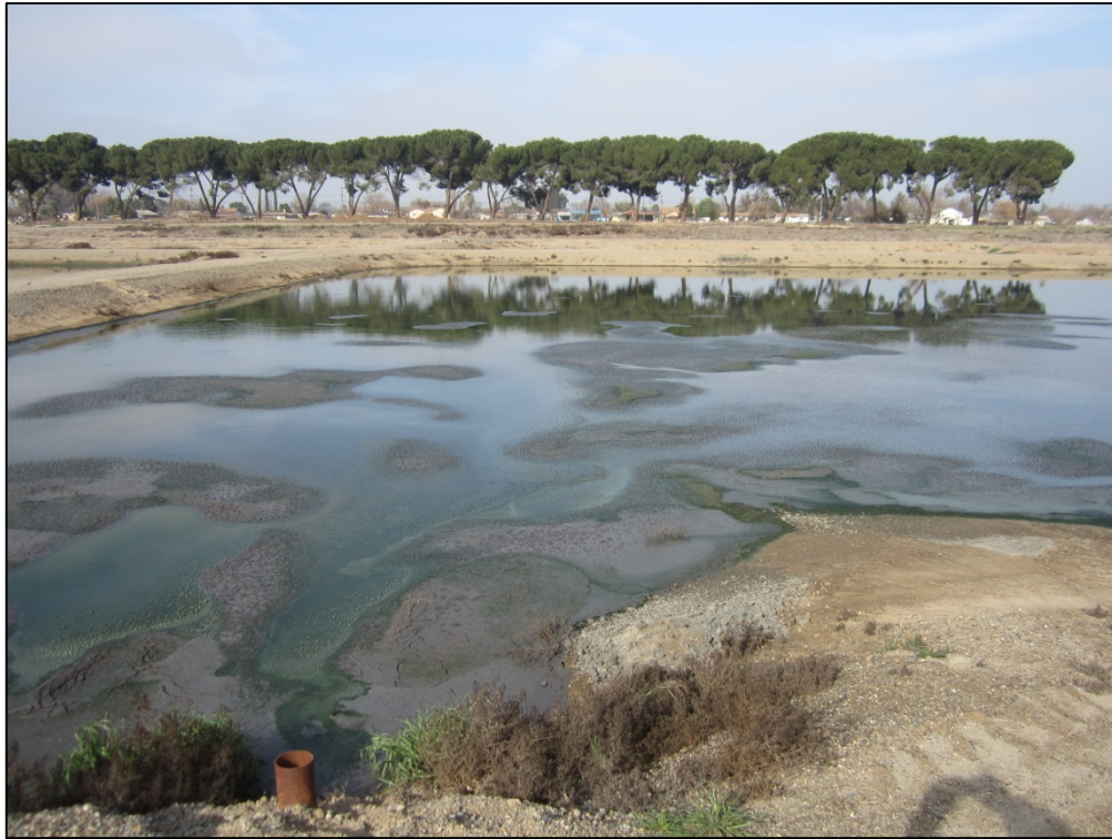
Figure 3-19 Sludge Drying Beds
