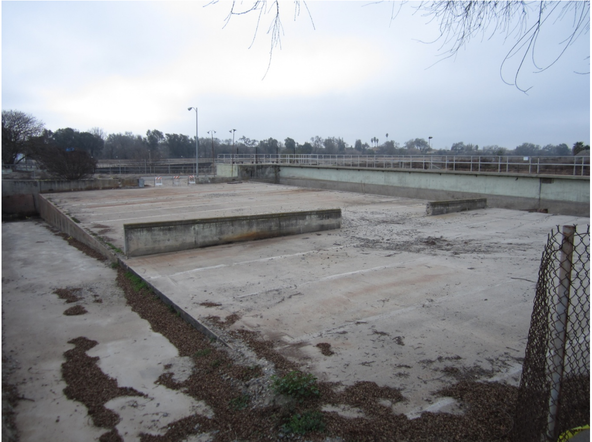
Figure 3-17 Aeration Structure converted to a Vac Con Truck unloading station
