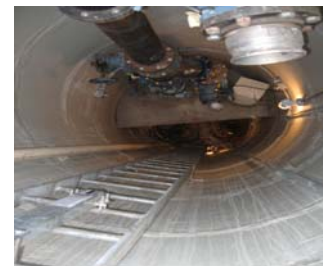
Hahn Lift Station Drywell
